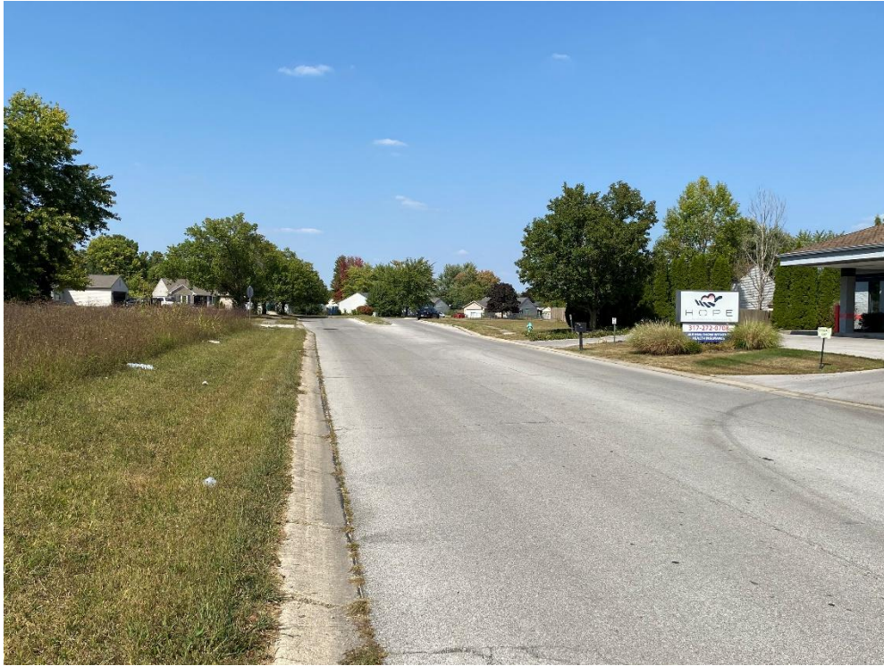
3) Facing north along Park Place Boulevard from front of site.
