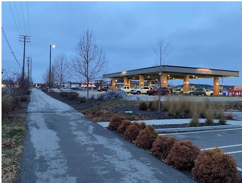
2) Facing west from front of site toward pedestrian walkway from U.S. 36.
