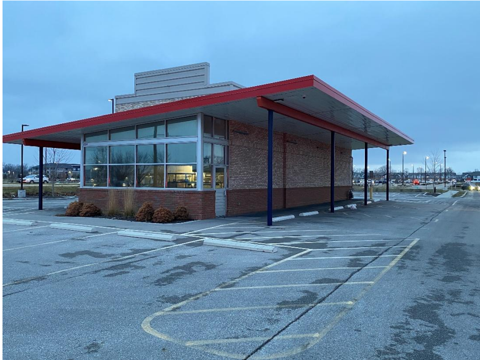
3) South and east façades of building.
