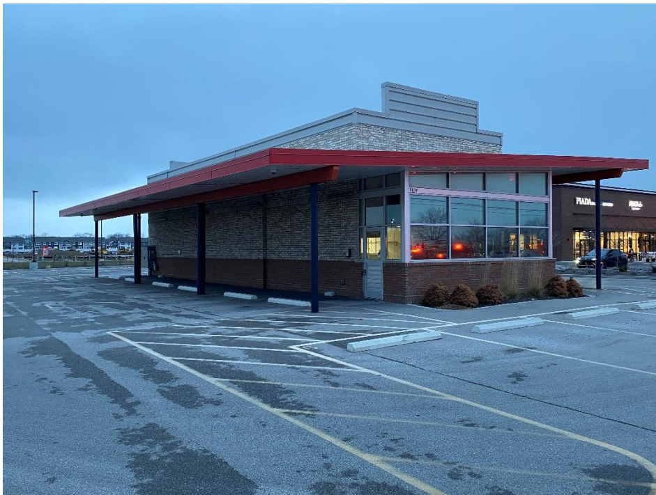
4) South and west façades of building.
